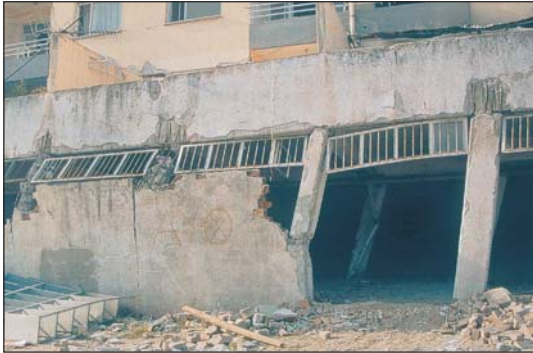
RIGHT: Damage to columns due to long openings & windows located at the edge of the column (Northridge, California 1994)
